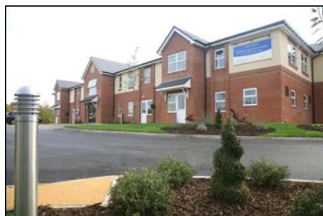
Christie + Co recently sold this Sheffield turn-key care home to Sanctuary Group.
